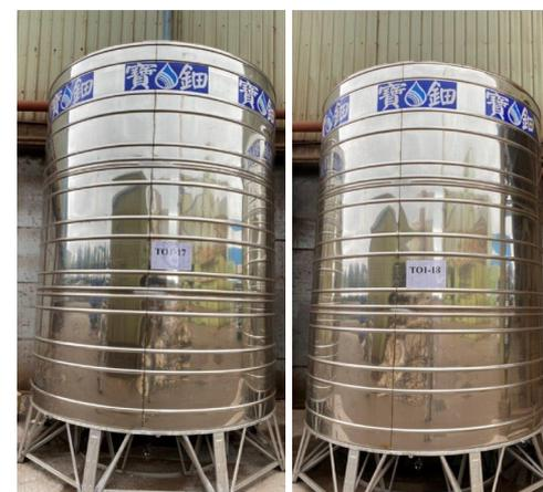
Water saving plan with new addition of 2 units of water reclamation tank with total of 20 tons for aggregation process
